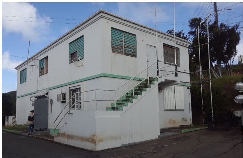
Pictured: VITEMA Emergency Operation Center on St. John.
